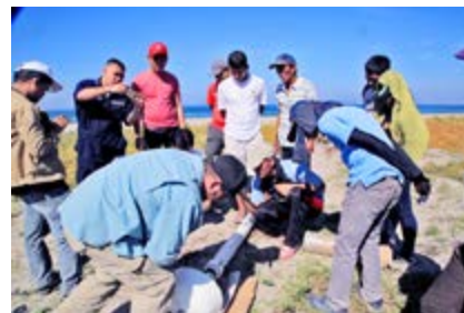
Final installation and erection of receiver and transmitter antennas
