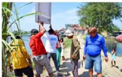
Installation of signage at Bulacan led by GMMA-READY Team
