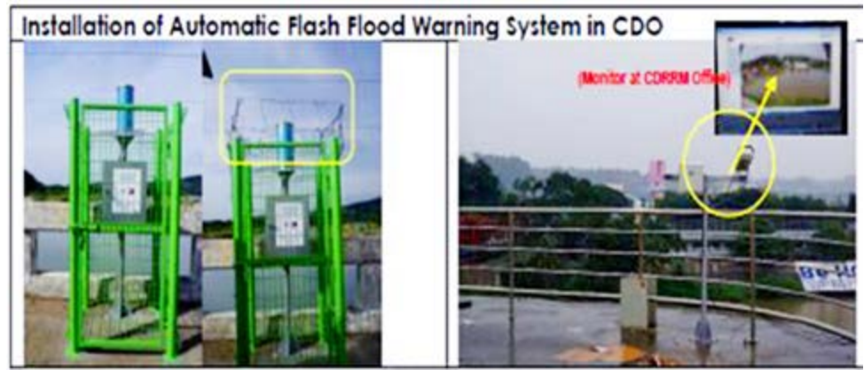
Barb wires were added at the installed ARG at Pelaez Bridge for better protection (left photo). Intelligent CCTV that can measure water level changes installed at the rooftop of the CDO City Hall Annex. (right photo)
