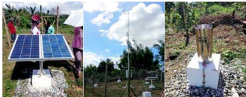
AWS, Installed in Mina, Iloilo under the PhilCCAP Project
