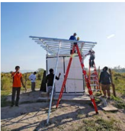
Re-alignment of Solar Panel Mounting Bracket at NETC
