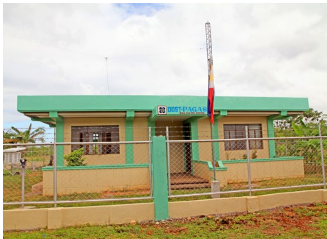
Newly constructed Dauis PAGASA Station
