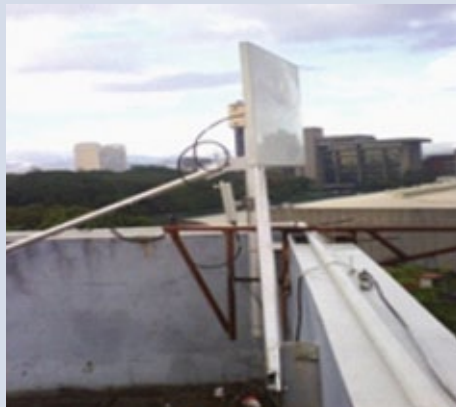
Broadband equipment installed at PAGASA-Telof site, Tagaytay; the system currently supports Tagaytay of NAIA-DIC link
