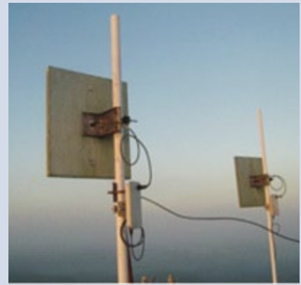
Broadband equipment installed at PAGASA-Telof site, Tagaytay; the system currently supports Tagaytay of NAIA-DIC link
