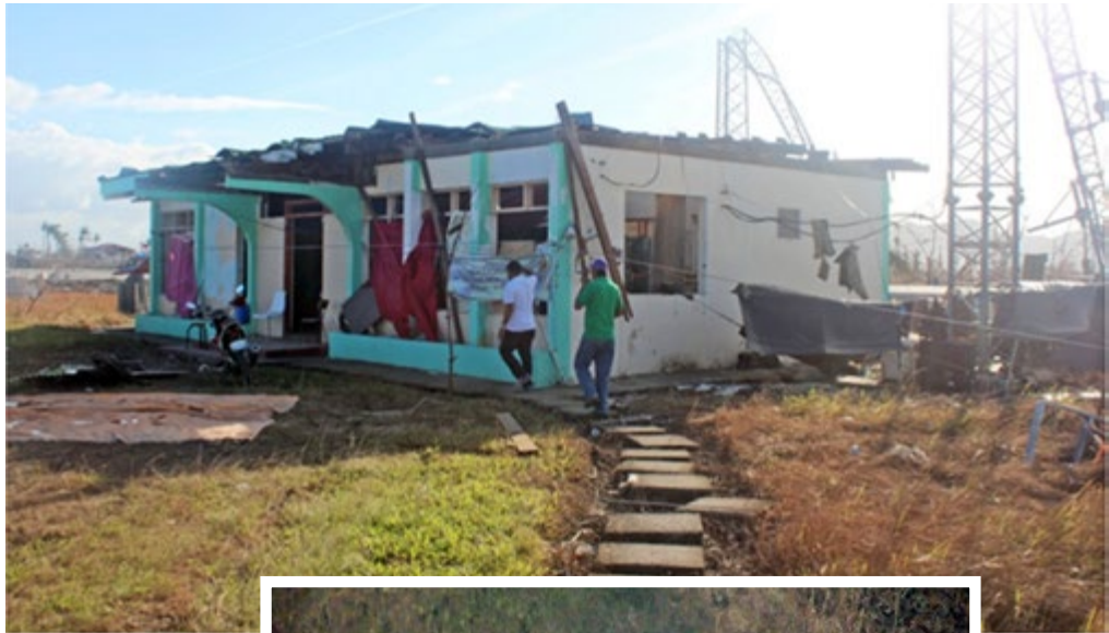
PAGASA Tacloban synoptic station after Typhoon Yolanda
