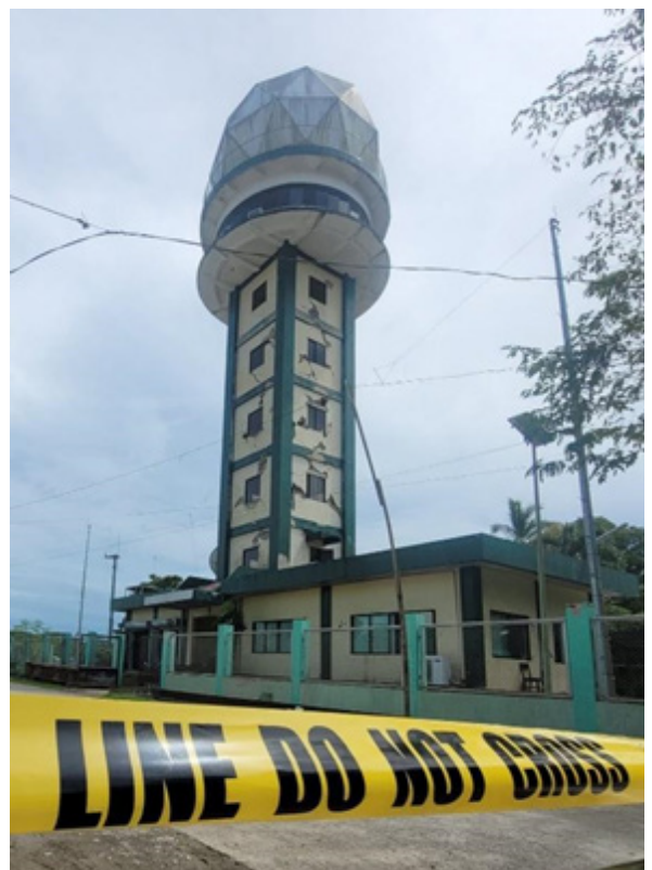
Hinatuan Synoptic and Radar Station after the earthquake
