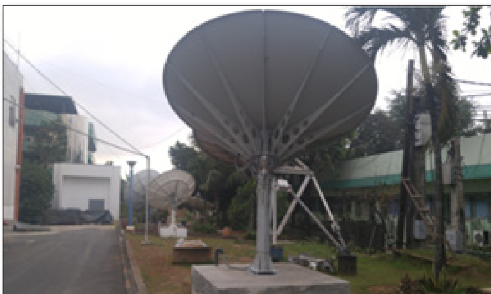
The COMS Antenna at Weather and Flood Forecasting Center
