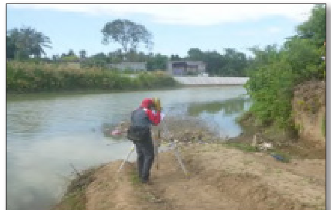
Conduct of river survey
