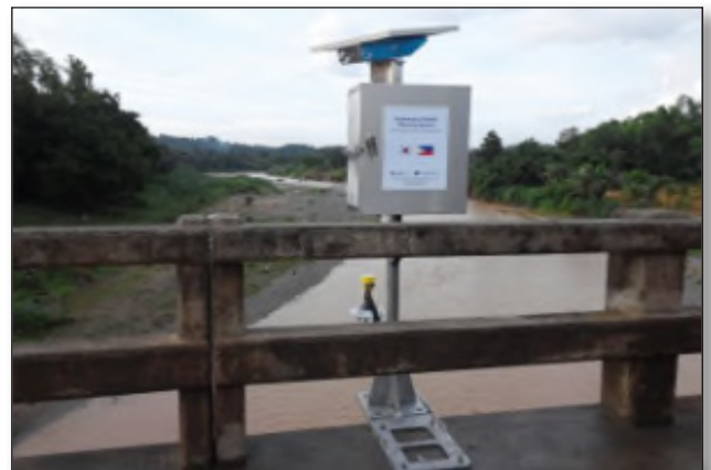
Water level observation system installed at San Simon Bridge, Iponan River Basin
