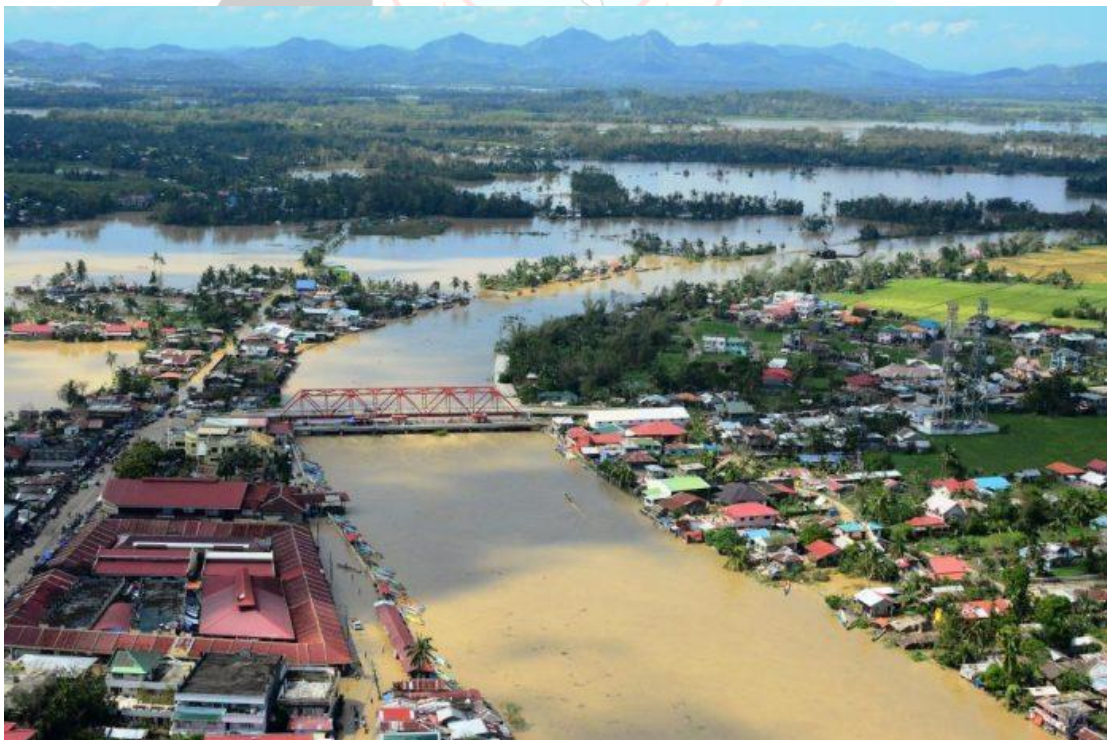
Fig 5.2.8. Aerial survey image of downtown Pontevedra in Capiz showing the extent of river flooding in the areas near the Panay River. Photo courtesy of Panay News (2019) contributor.
